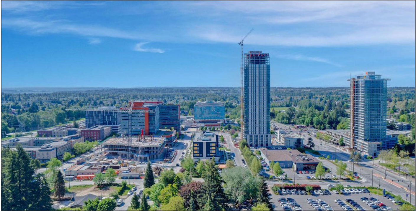
City Centre 4 beginning to rise (left), Comma King George (centre), and Belvedere (right)
