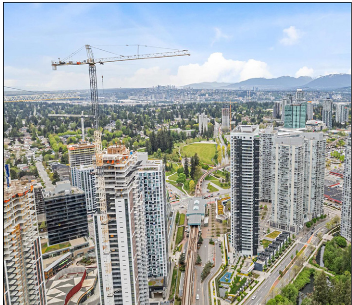
Plaza One & Two topping out at King George Hub
